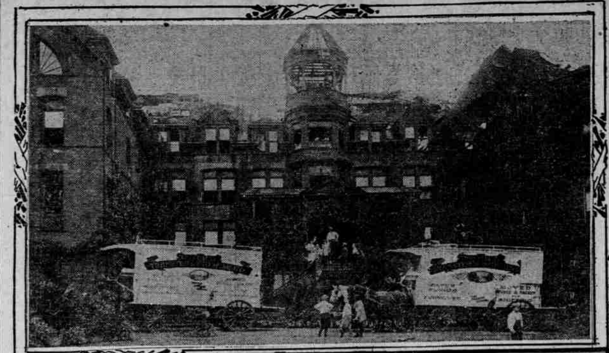
Damage Done by The Flames
