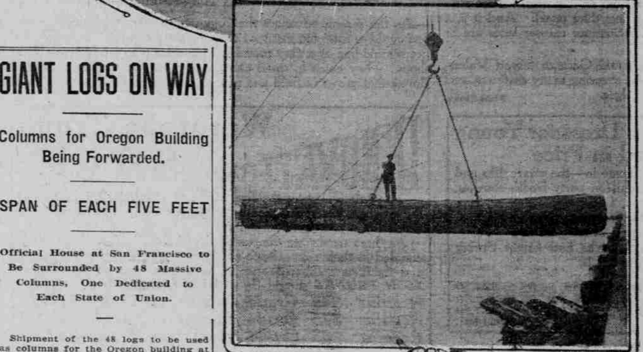
Top—Loading Cars at Albina Dock With Logs Weighing 25,000 Pounds Each. Middle—Log Being Lowered at Albina Dock by Only Derrick in Northwest That Can Handle Them. Bottom—Derrick Raising Log Out of Boat to Flatcar.
