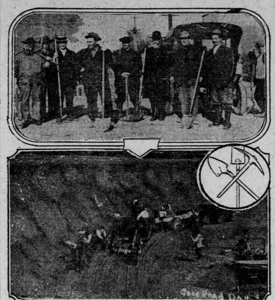
TOP—PICK AND SHOVEL SQUAD READY FOR WORK.—BELOW—SCENE IN GRAVEL PIT.
