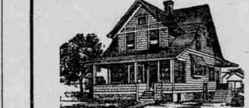
A No. 1, 22-W IDEAL Boiler and 400 ft. of 38-IN. AMERICAN Radiators costing the owner $190, were used to heat this cottage. At this price the goods can be bought of any reputable, competent fitter. This did not include costs of labor, pipe, valves, freight, etc., which are extra and vary according to climatic and other conditions.
