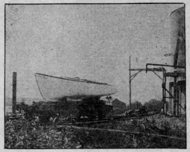
CRAFT EQUIPPED WITH AUTOMOBILE CONTROL The Alert of Clatskanie was constructed by Williard T. and Frank-lin Evenson, sons of O. J. Evenson, manager of the Benson Timber Com-pany. The boat is 32 feet in length and beam of 4 feet 8 inches. It
