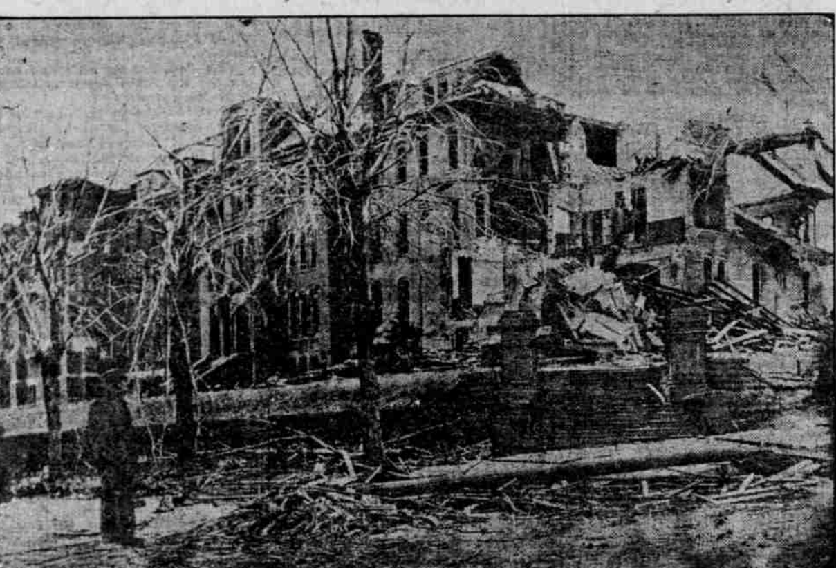
ABOVE—VIEW OF DAMAGE IN NEGRO SECTION. BELOW—WRECK OF SACRED HEART HOSPITAL.
