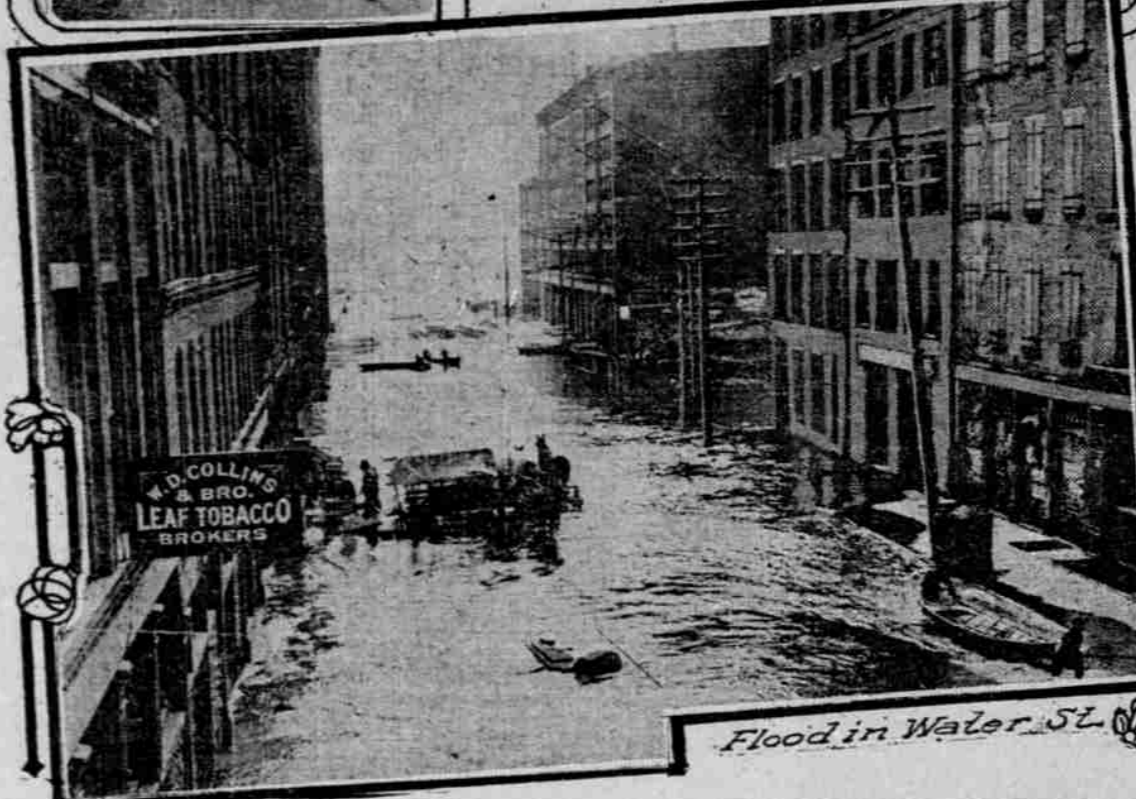
Flood in Water St.
