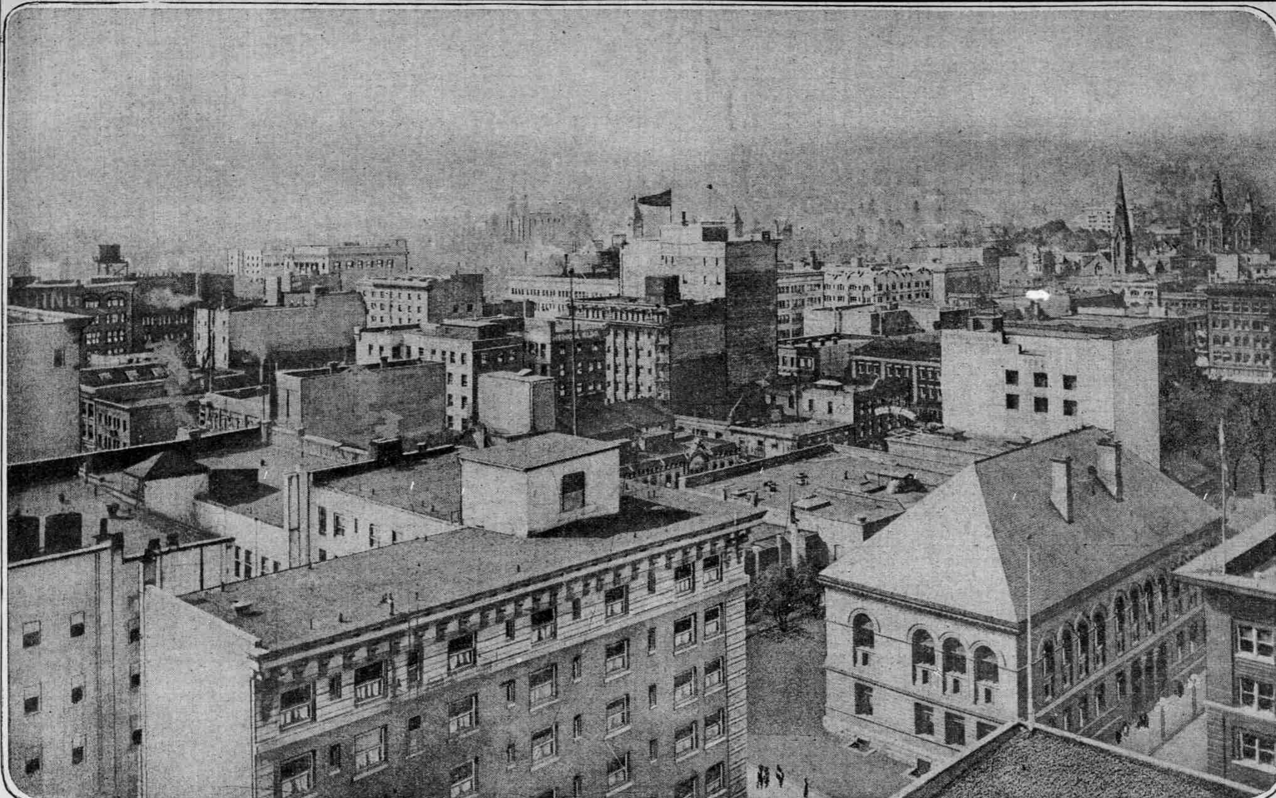
Western Section Of Business District, Looking South-West From Wells-Fargo Building.
