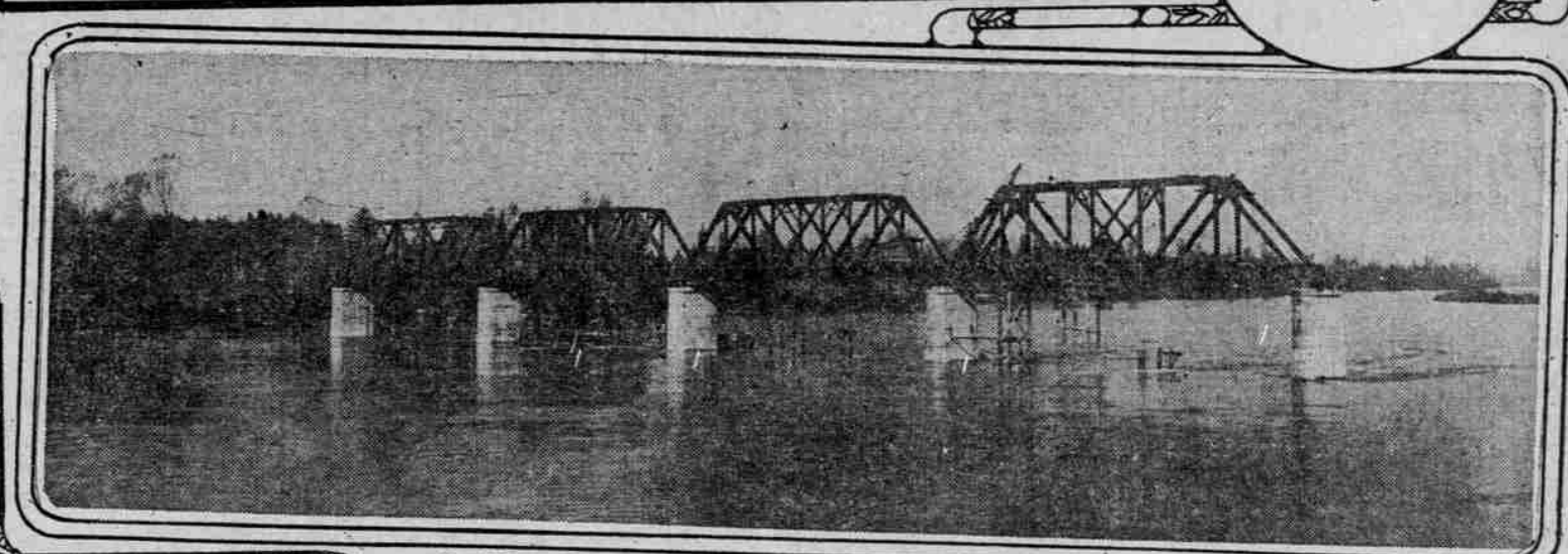
Bridge Over Willamette River At Salem, Nearing Completion.
