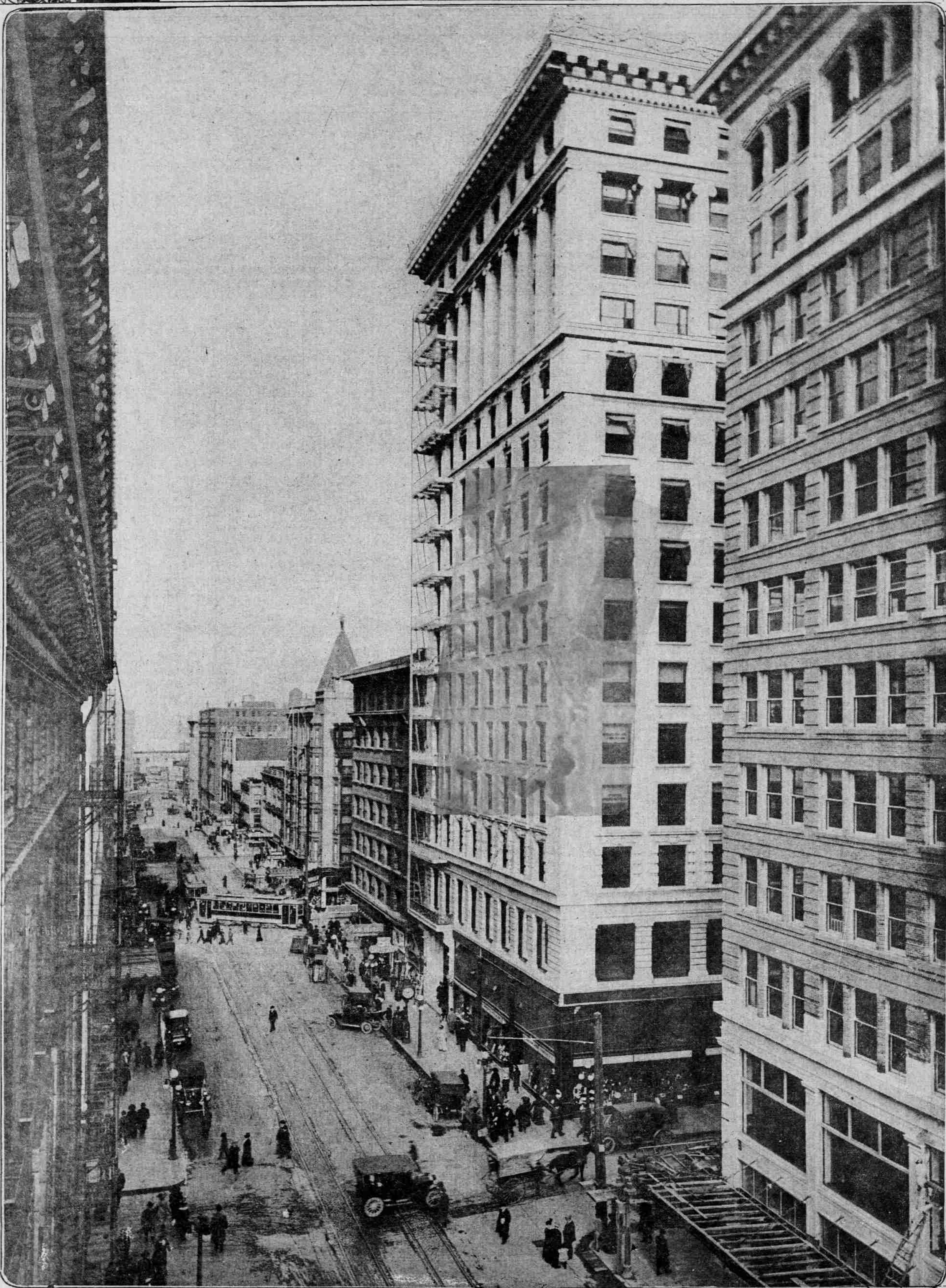
FIFTH STREET NORTH FROM ALDER.
