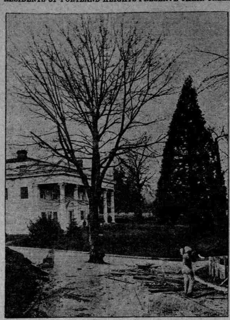
FINE MAPLE LEFT STANDING IN MIDDLE OF PAVED STREET.
