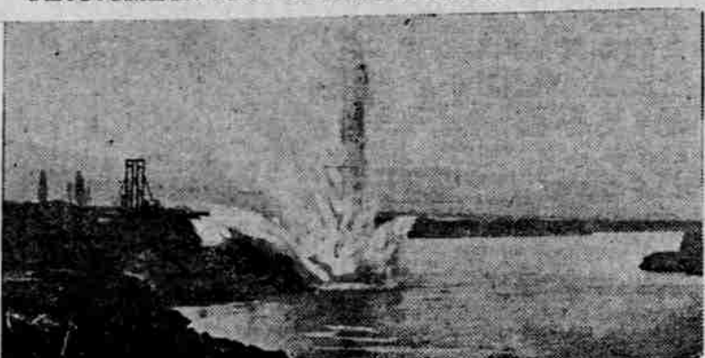
BLASTING ROCKS FROM RIVER BED.
