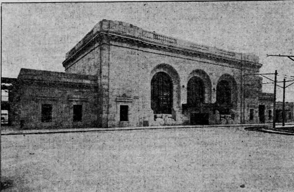
STRUCTURE, WHICH COST $350,000, HAS TWO TRACK LEVELS—FOR STEAM AND ELECTRIC TRAINS.
