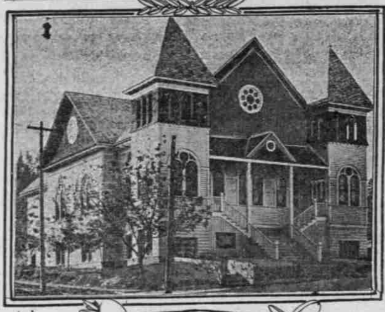
ABOVE, NEW HIGH SCHOOL BUILDING—CENTER, PRESBYTERIAN CHURCH—BELOW, SHEEP GRAZING IN FOREST RESERVE.
