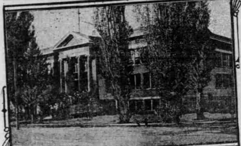
$50,000 HIGH SCHOOL BLDG. JUST COMPLETED AT UNION, ONE OF THE FINEST IN THE STATE.
