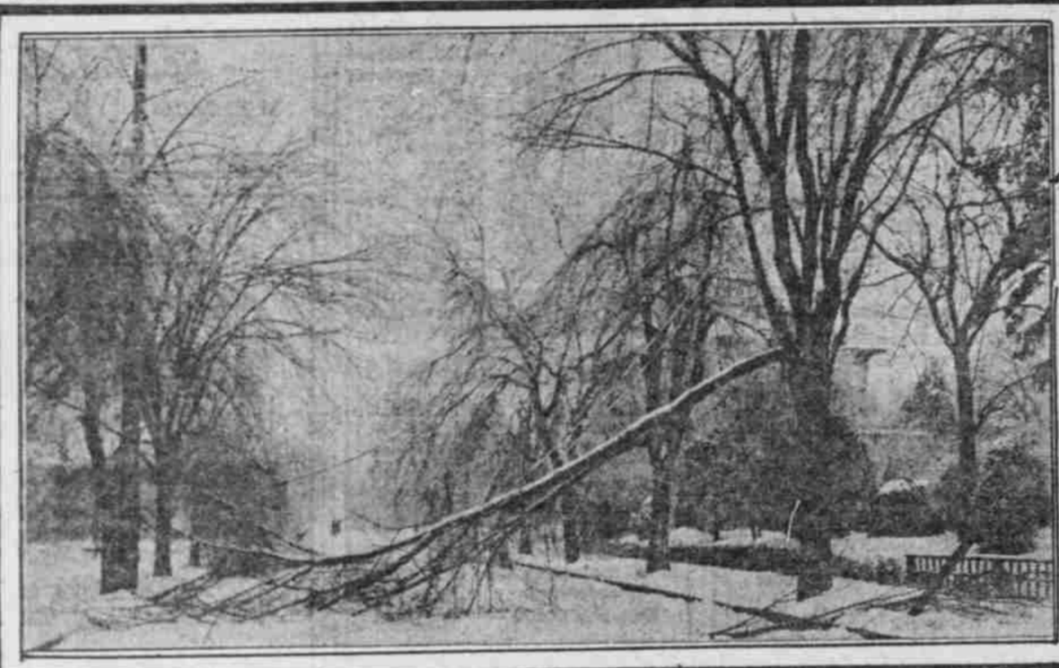
VISTA ON KEARNEY ST. BETWEEN 20th AND 21st STS.
