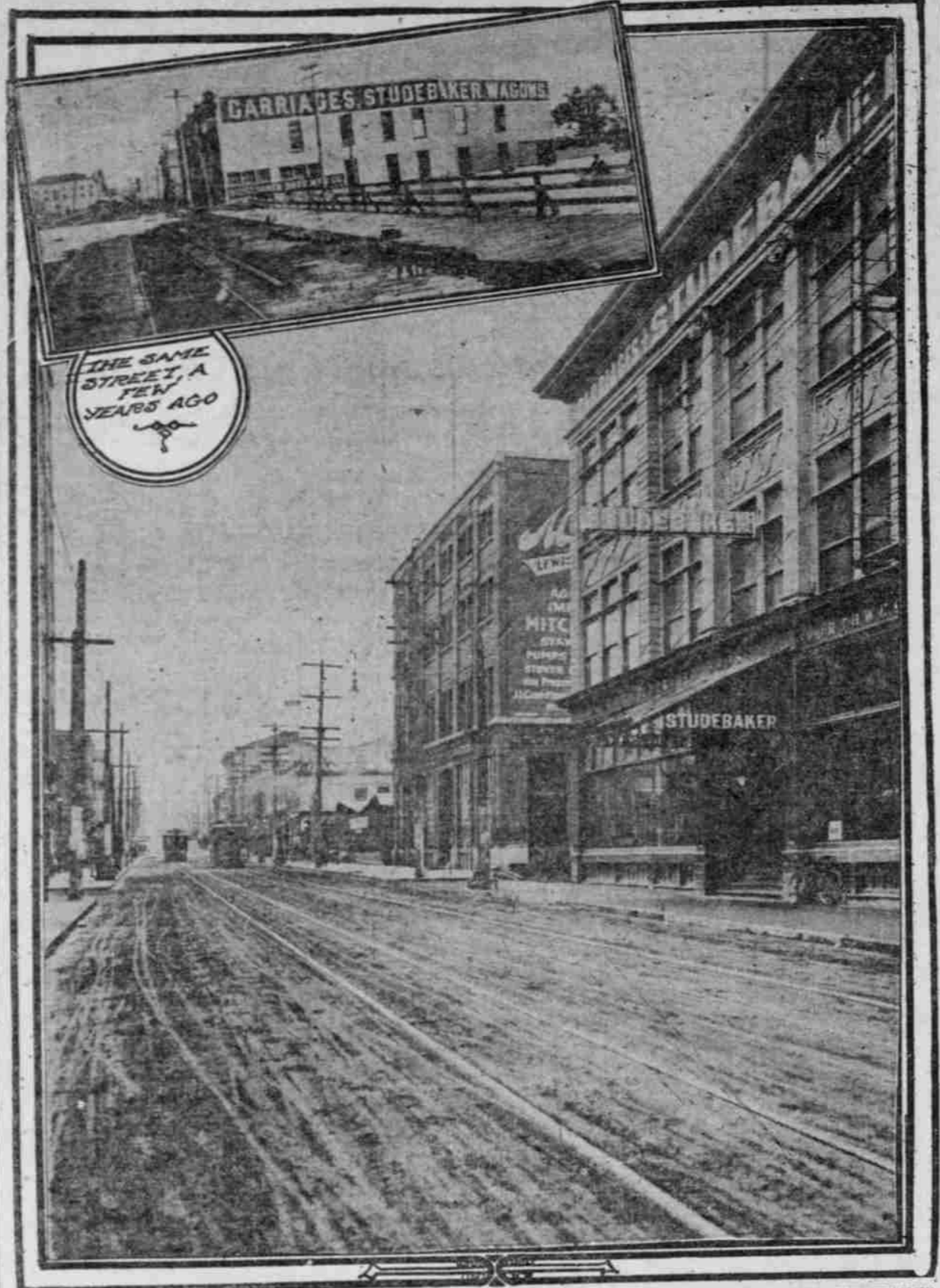
PLANKS GIVE WAY TO CARBOLINEUM-TREATED WOOD BLOCKS, LAID IN RECORD TIME BY FISHER, THORSEN & COMPANY. THIS BRAND OF PAVEMENT HAS COST THE CITY NOTHING FOR MAINTENANCE IN PAST 11 YEARS.
