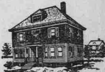
A No. 17-3-W IDEAL Boiler and 300 ft. of 38-in. AMERICAN Radiators, costing the owner $148, were used to heat this cottage. At this price the goods can be bought of any reputable, competent Fitter. This did not include cost of labor, pipe, valves, freight, etc., which are extra and vary according to climatic and other conditions.
