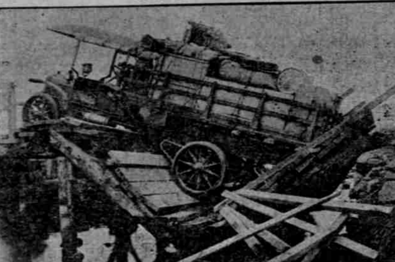
MACHINE WHICH BROKE DOWN BRIDGE.
