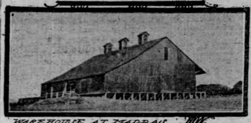
WAREHOUSE AT MADRAS.
