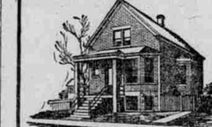
No. C-118 IDEAL Boiler and 270 ft. of 38-in. AMERICAN Radiators, costing over $135, were used to heat this cottage. At this price, the goods can be bought of any reputable, competent fitter. This did not include cost of labor, pipes, valves, fittings, etc., which install in extra and varies according to climatic and other conditions.
