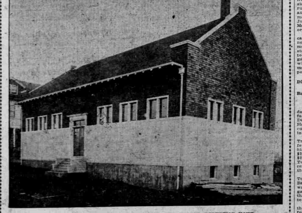
GYMNASIUM AND MANUAL TRAININGSHOP OF THE FRAZER DETENTION HOME.
