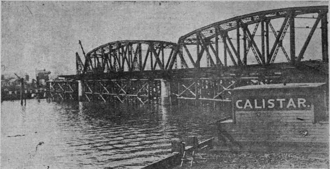
MADISON-STREET CROSSING OVER WILLAMETTE RIVER AS IT APPEARS TODAY.
