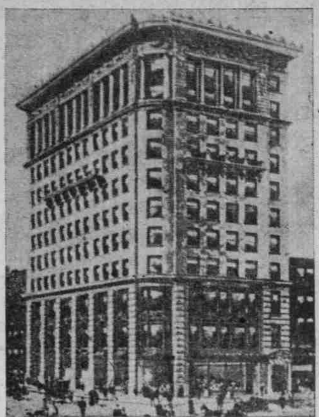
Office Building, Fifth Ave., N. Y. No Fire Escapes.
