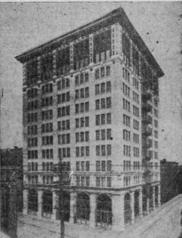
Wells Fargo Bldg., Portland, 12 Stories, One Fire Escape.
