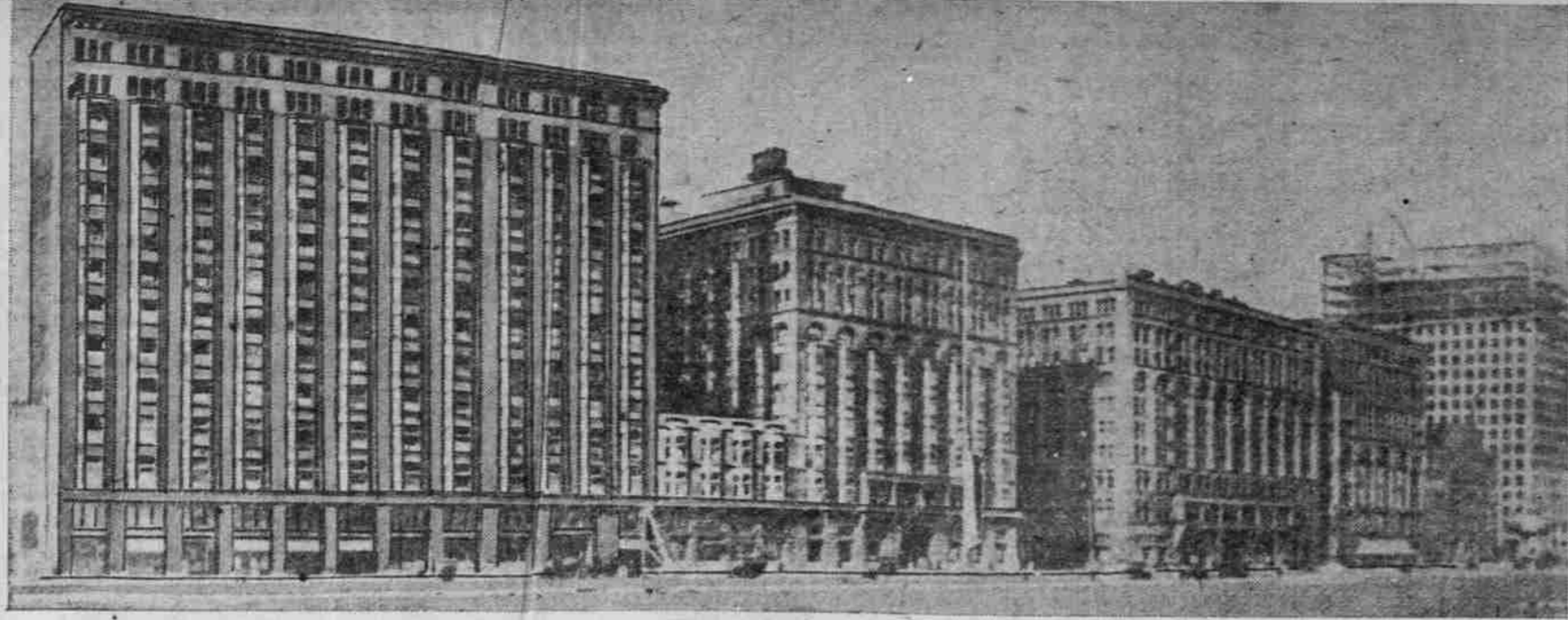
71 1/2 Boulevard, Chicago. No Fire Escapes.
