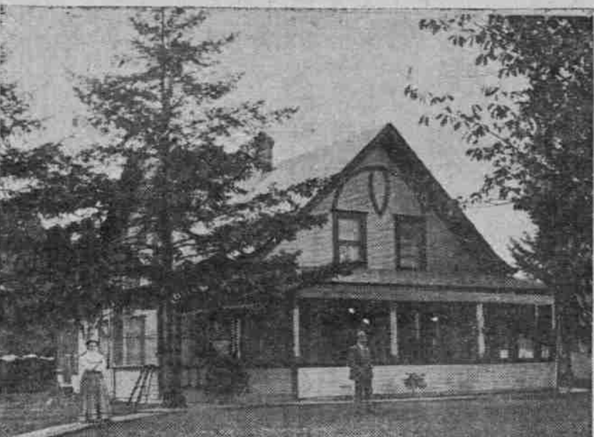
RESIDENCE OF O. M. KERN.
