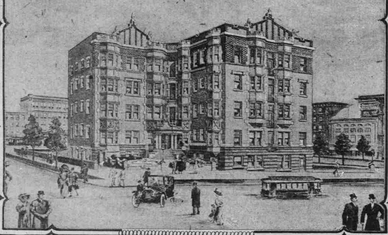
SUNNYSIDE APARTMENTS UNDER CONSTRUCTION LUCRETIA ST. NEAR WASHINGTON ST.
