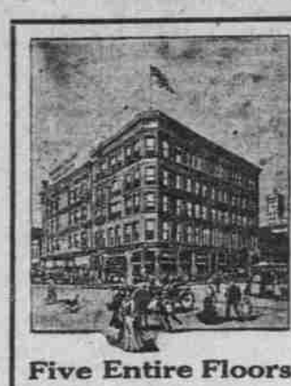
Five Entire Floors
