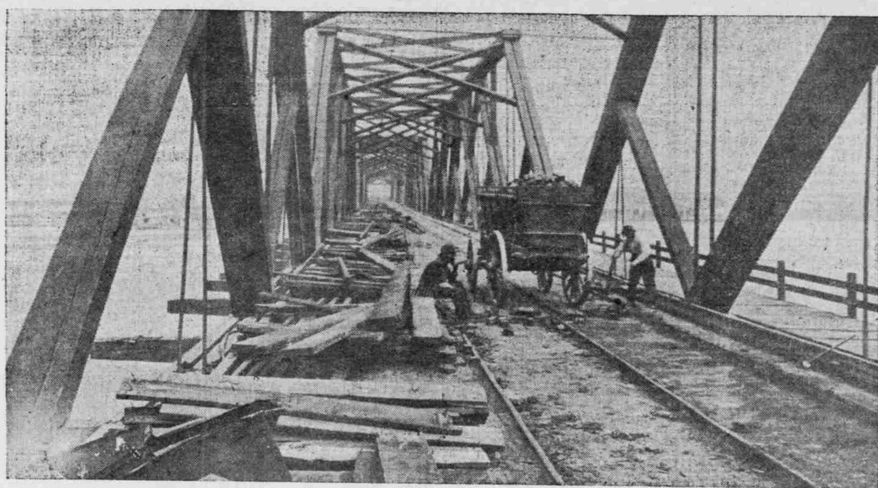
HAULING OFF OLD WOOD BLOCK PAVEMENT FROM DECK OF SPAN.
