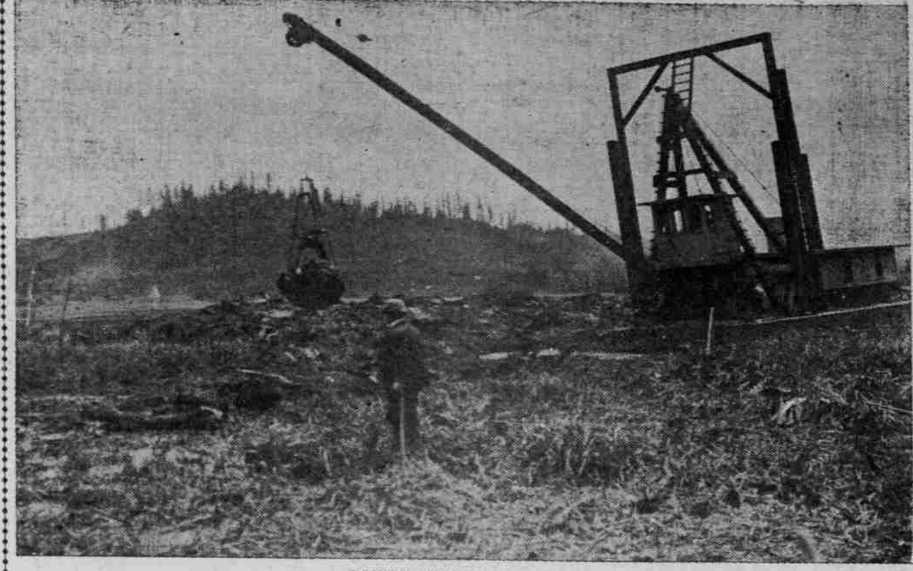
POWER-SHOVEL IN ACTION.
