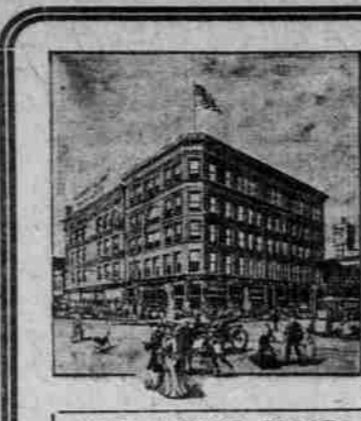
FIVE ENTIRE FLOORS.
