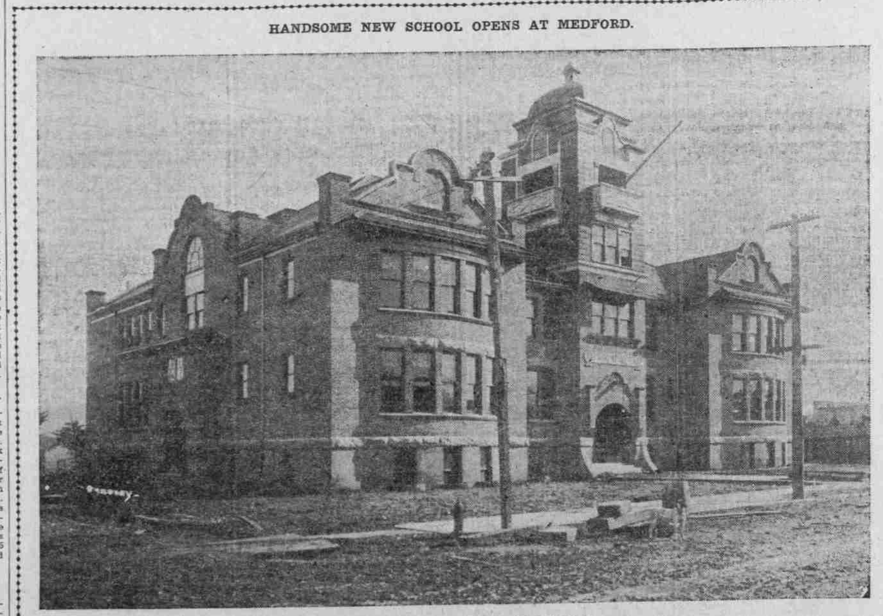
HANDSOME NEW SCHOOL OPENS AT MEDFORD. MEDFORD, Or., Feb. 14.—(Special.)—Medford's new High School building, which has just been completed at a cost of $40,000, will be occupied for the first time tomorrow. The building is a modern in every respect, contains nine large recitation rooms, large laboratory and auditorium said to be the finest in any school building in the state. The dedication exercises will be held in the building April 9.
