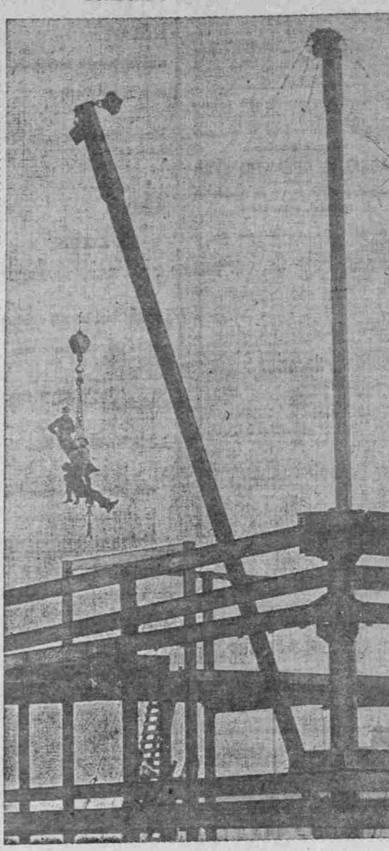
FREQUENT RISKS TAKEN BY SKILLED MECHANICS ATTRACT MUCH ATTENTION.
