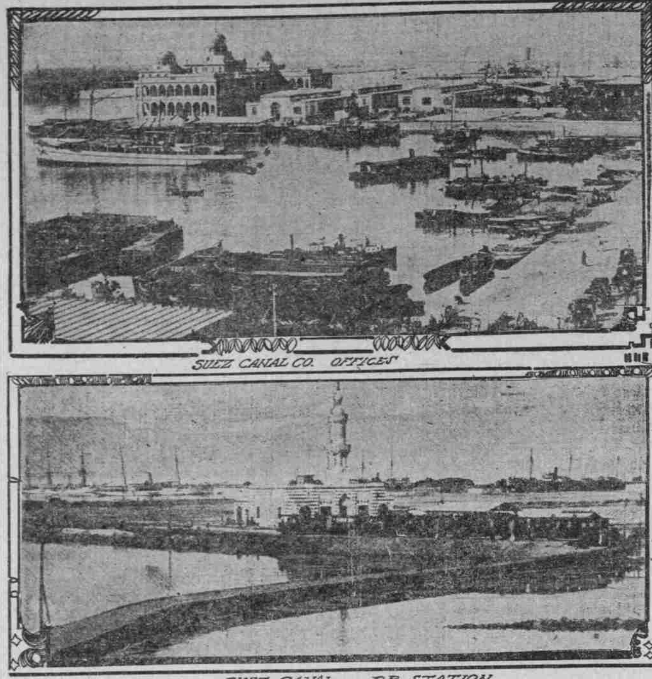
SUEZ CANAL - RR STATION.
