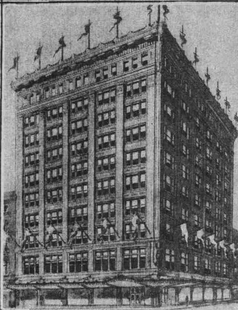
MEIER AND FRANK COMPANY'S TEN-STORY ANNEX NOW UNDER CONSTRUCTION
