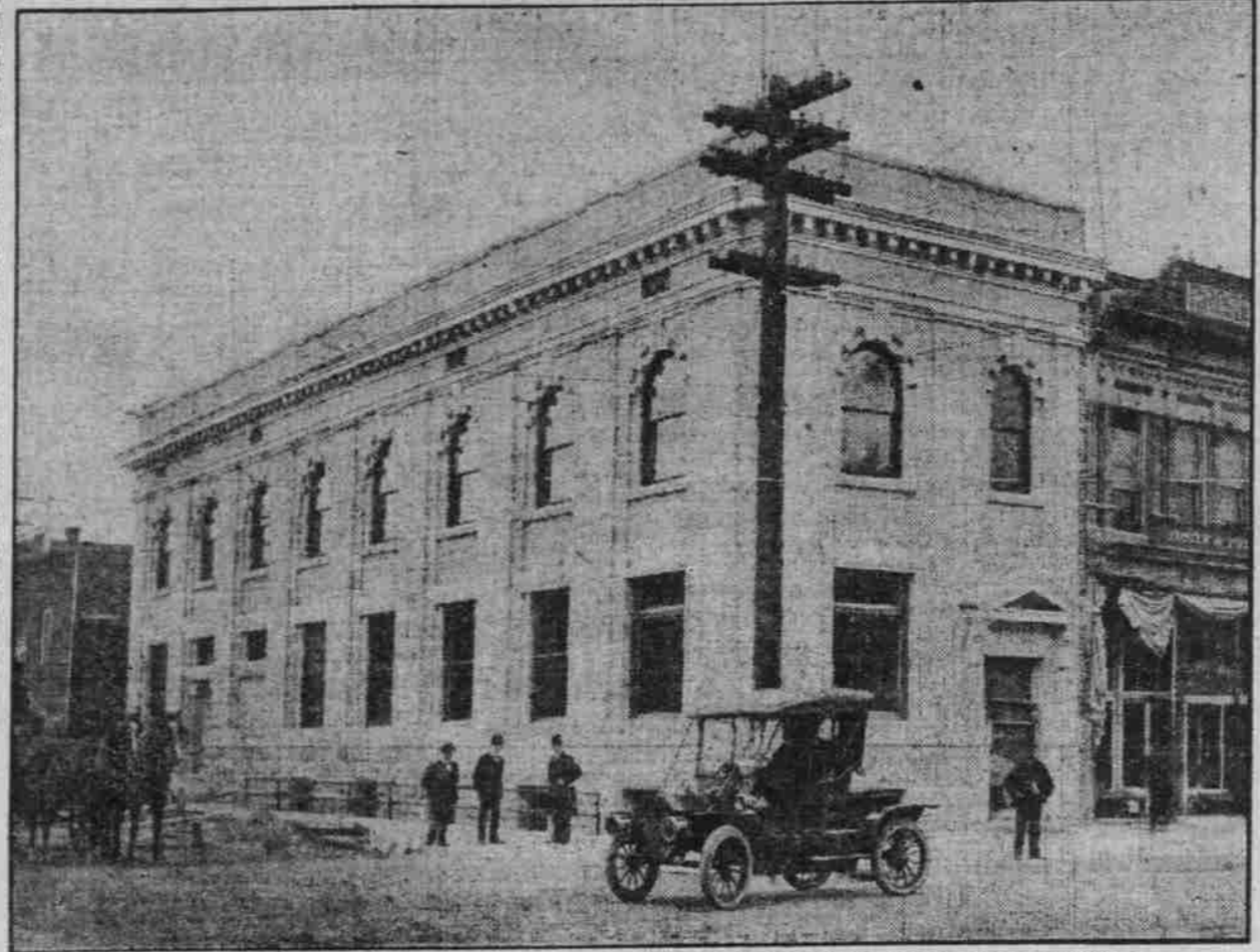
FUTURE HOME OF CITIZEN'S NATIONAL BANK, TO COST WHEN COMPLETED $50,000.
