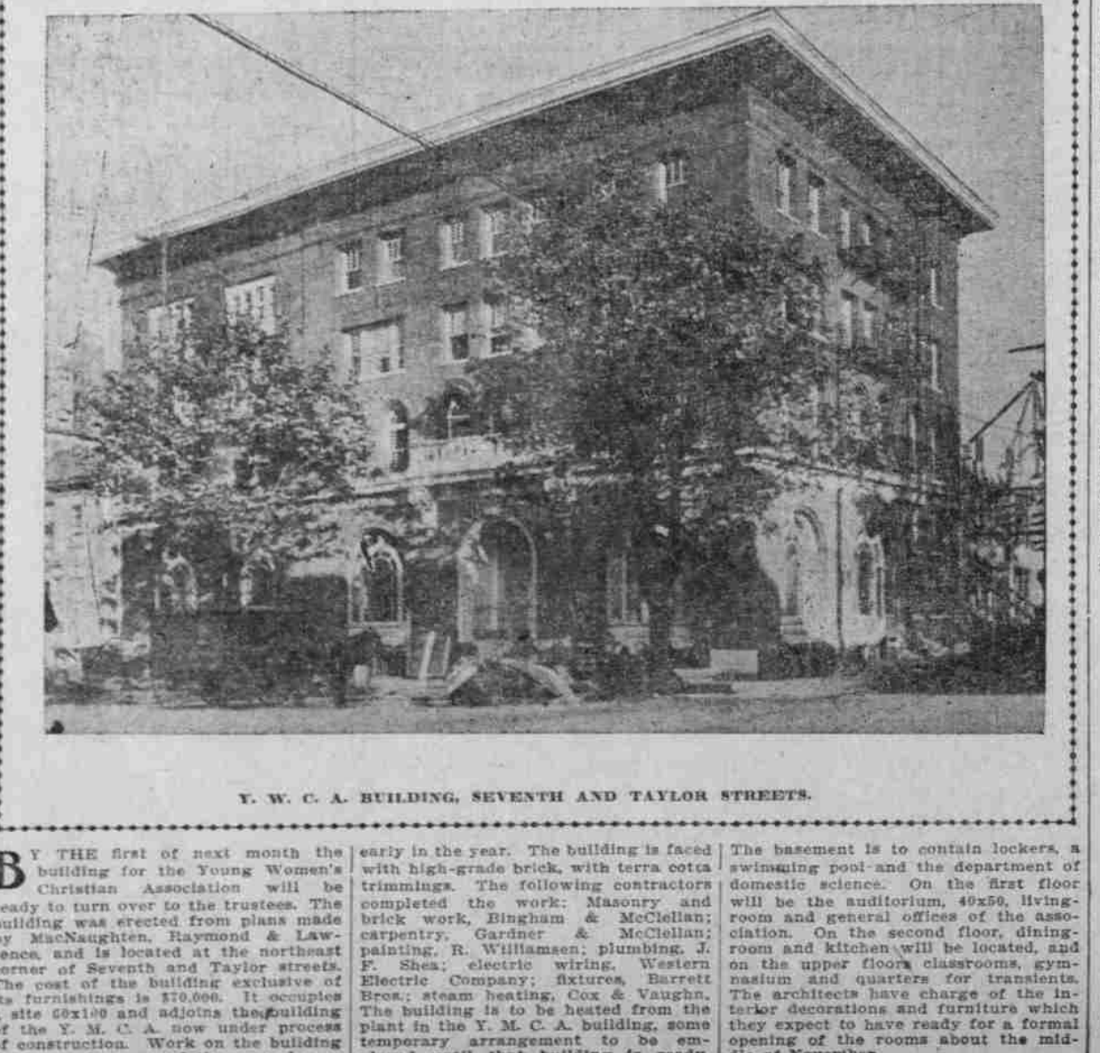
Y. W. C. A. BUILDING, SEVENTH AND TAYLOR STREETS.
