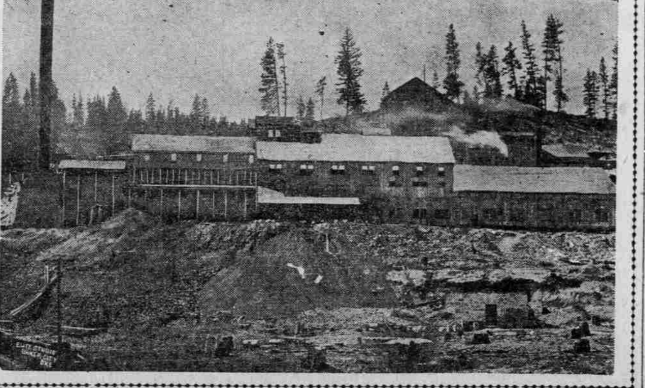
SMELTER IN BAKER COUNTY THAT WILL HANDLE ORE SHIPPED IN OVER NEW EAGLE VALLEY RAILROAD
