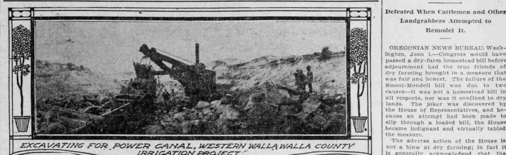
EXCAVATING FOR POWER CANAL, WESTERN WALLA WALLA COUNTY IRRIGATION PROJECT
