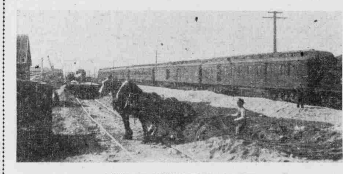
LAYING NEW RAILROAD TRACKS AT EUGENE.
