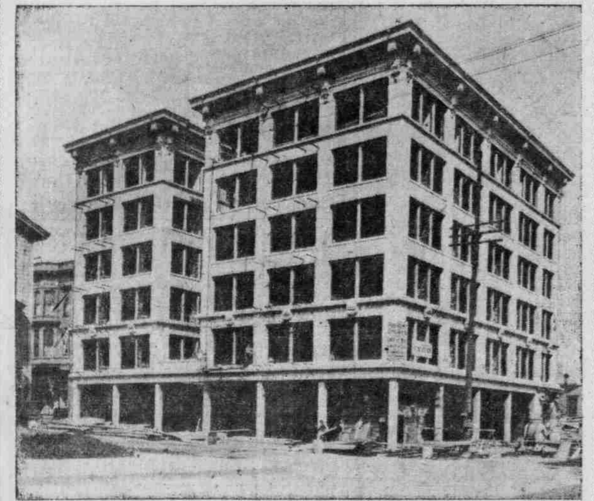
THE BECK BUILDING, NEARING COMPLETION, CORNER SEVENTH AND OAK STREETS.
