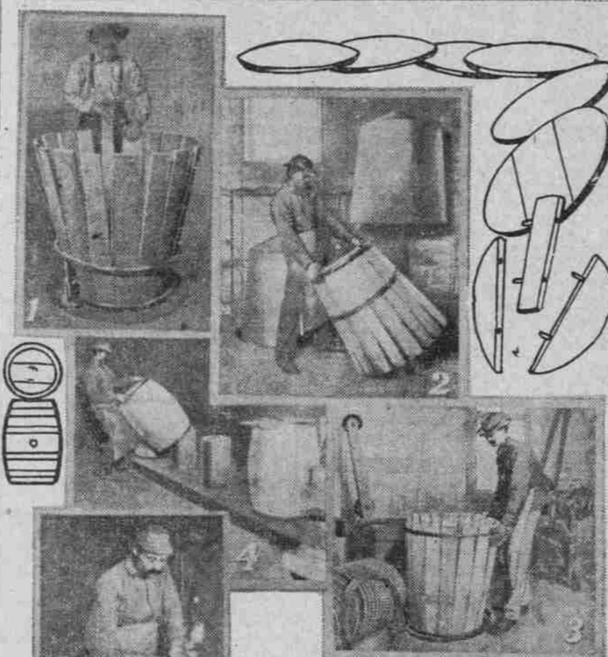
FIG. 5—MAKING THE BARREL
