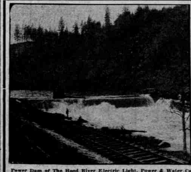
Power Dam of The Hood River Electric Light, Power & Water Co. Showing Waste Gate and Intake at Upper End of Pipe Line.
