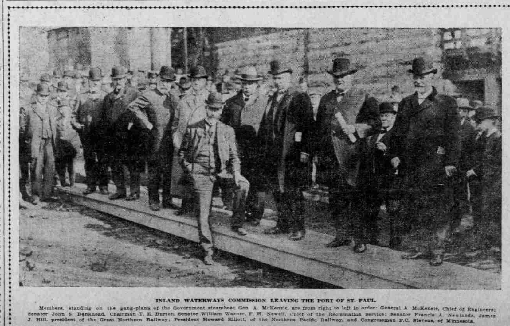
INLAND WATERWAYS COMMISSION LEAVING THE PORT OF ST. PAUL. Members standing on the gang-plank of the Government steamboat Gen. A. McKenzie, are from right to left in order: General A. McKenzie, Chief of Engineers; Senator John S. Bankhead, Chairman T. B. Burton, Senator William Garner, F. H. Newell, Chief of the Reclamation Service; Senator Francis A. Newlands, James J. Hill, president of the Great Northern Railway; President Howard Elliott of the Northern Pacific Railway; and Congressman F. C. Stevens, of Minnesota.
