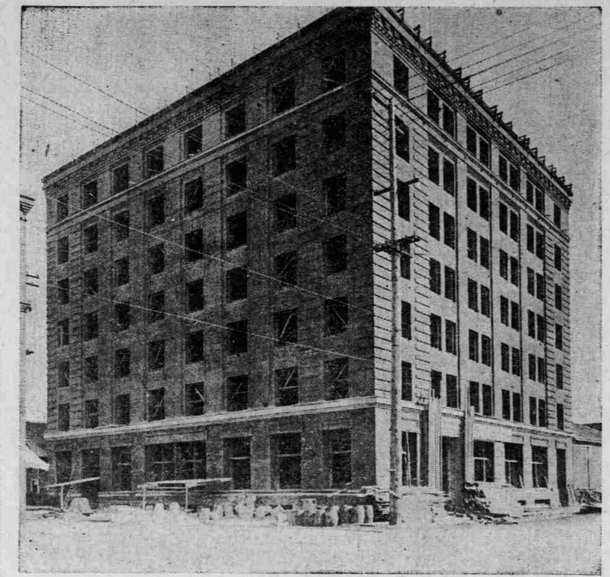
BUILDING ERRECTED FOR MASON, EHRMAN & COMPANY AT FIFTH AND EVERETT STREETS. One of the finest wholesale houses to be erected in Portland this year is the seven-story block for Mason, Ehrman & Company at Fifth and Everett streets. The construction of this building marks the extension of the wholesale district northward, many indications of which have been seen during the past few months. This building is seven stories in height and one of the best-constructed warehouses in the city. Workmen are now busy on the interior construction.
