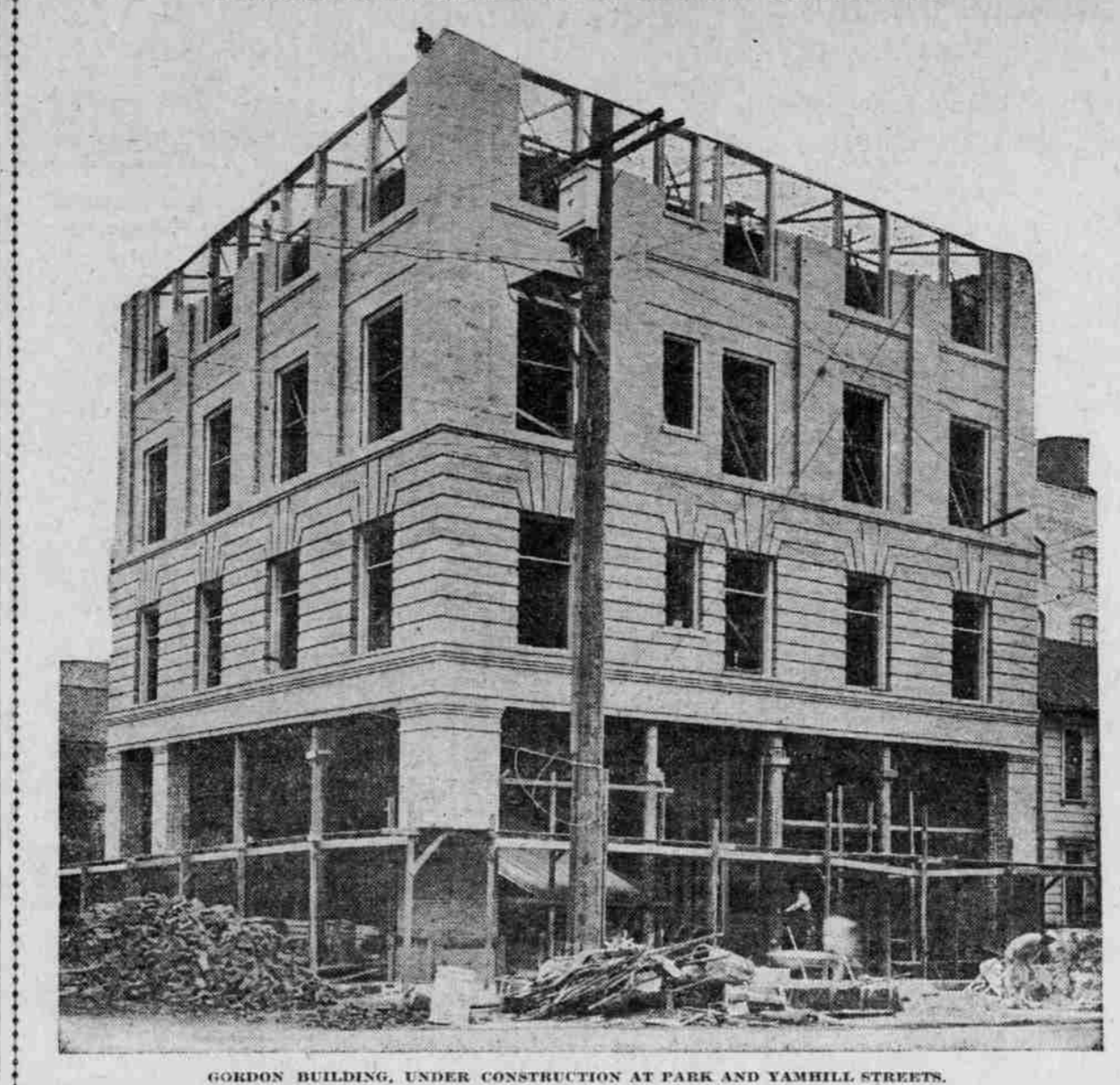
GORDON BUILDING, UNDER CONSTRUCTION AT PARK AND YAMHILL STREETS.
