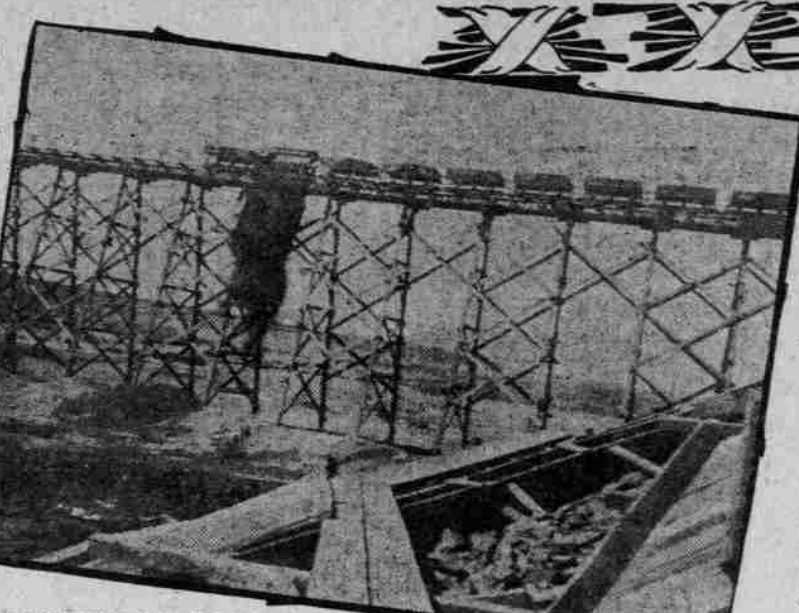
TRESTLE, COLD SPRINGS DAM SHOWING DUMP CARS AT WORK
