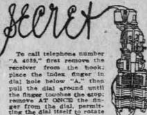
the finger touches the stop; remove AT ONCE the fin-ger from the dial, permit-ting the dial itself to rotate until it stops. Do not FORCE it back. In the
