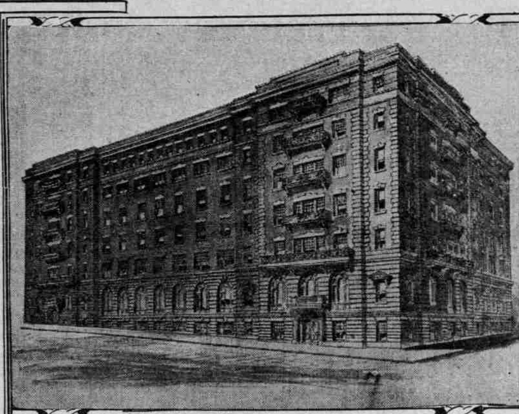
Y.M.C.A. BUILDING TO BE ERECTED DURING 1907
