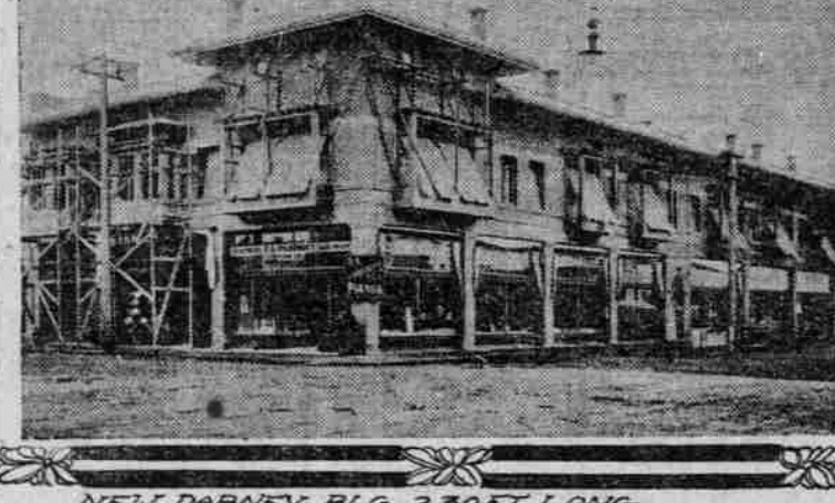
NEW DABNEY BLDG., 230 FT. LONG, CORNER G. AND WISHKAH ST., ABERDEEN
