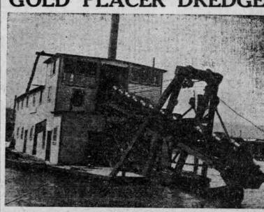
The Hammond steam, friction-driven dredge, shown in above cut, is for sale at Portland, Or. Digging capacity 250 cu. yds. per day. Capacity of buckets 5 cu. ft. each. It is new throughout, has been given three weeks' continuous test and is a thoroughly up-to-date gold dredge. It may be purchased with or without the hull, and the superstructure may
